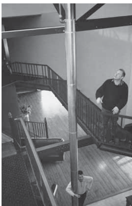
ABOVE L to R: Marshall booster - designed to heat water for heating systems - shown here in the basement of a 3-storey restaurant. The flue is completely surrounded in water, so no heat is wasted in just going up the chimney - it's heating water all the way up. The first floor branches off the flue for underfloor heating. CENTRE RIGHT: 150 gallon copper, uninsulated water heater - radiates heat to help warm the room as well as contain a large volume of hot water.
