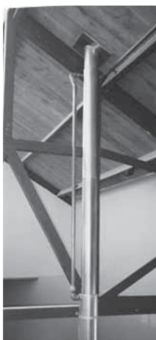
ABOVE L to R: Marshall booster - designed to heat water for heating systems - shown here in the basement of a 3-storey restaurant. The flue is completely surrounded in water, so no heat is wasted in just going up the chimney - it's heating water all the way up. The first floor branches off the flue for underfloor heating. CENTRE RIGHT: 150 gallon copper, uninsulated water heater - radiates heat to help warm the room as well as contain a large volume of hot water.
