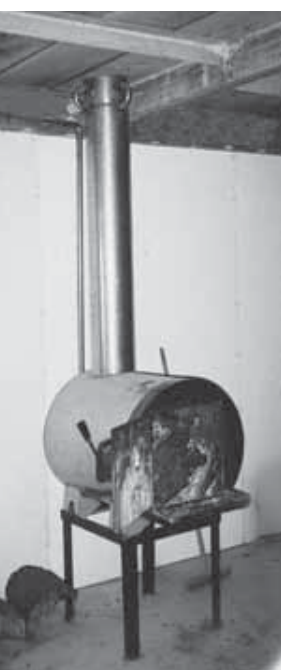
ABOVE L to R: Marshall booster - designed to heat water for heating systems - shown here in the basement of a 3-storey restaurant. The flue is completely surrounded in water, so no heat is wasted in just going up the chimney - it's heating water all the way up. The first floor branches off the flue for underfloor heating. CENTRE RIGHT: 150 gallon copper, uninsulated water heater - radiates heat to help warm the room as well as contain a large volume of hot water.
