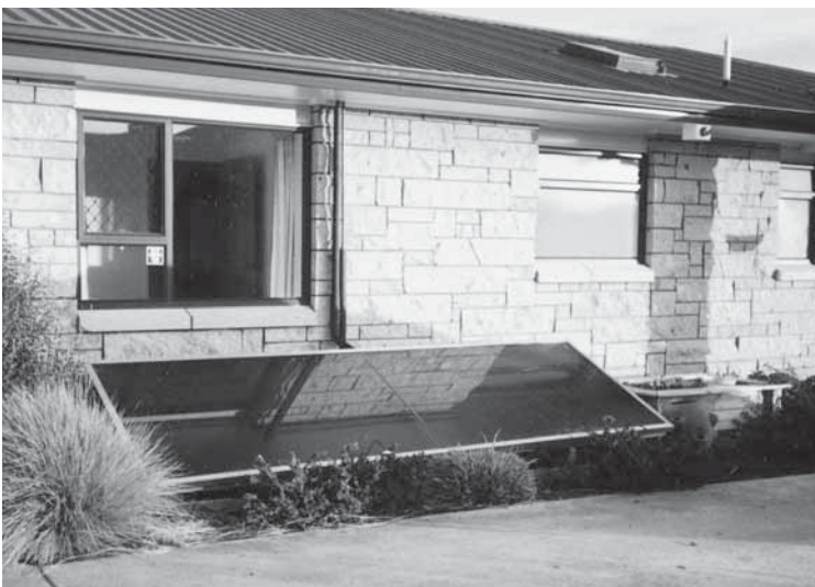
TOP LEFT: The Solar heater Henry designed 20 years ago. The entire surface collects the heat as opposed to copper pipes sitting on a collector plate. Seen here installed at ground level, and working on the thermo-syphoning system - no electric pumps required.
