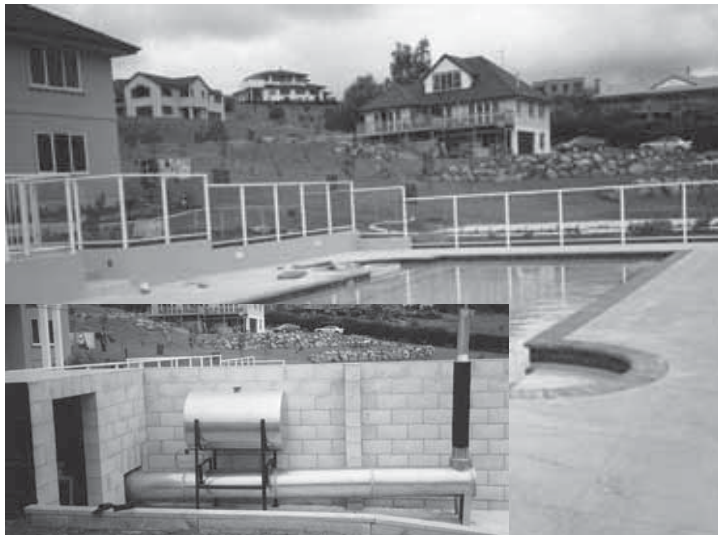
TOP LEFT: The Solar heater Henry designed 20 years ago. The entire surface collects the heat as opposed to copper pipes sitting on a collector plate. Seen here installed at ground level, and working on the thermo-syphoning system - no electric pumps required.
